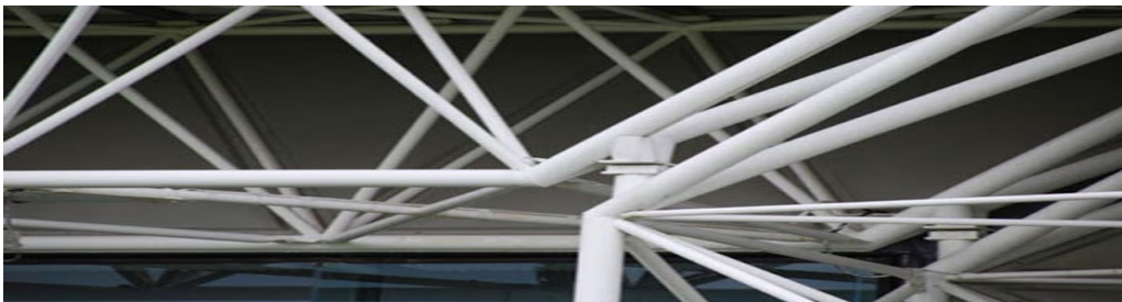
Figure 6. welding in joint
